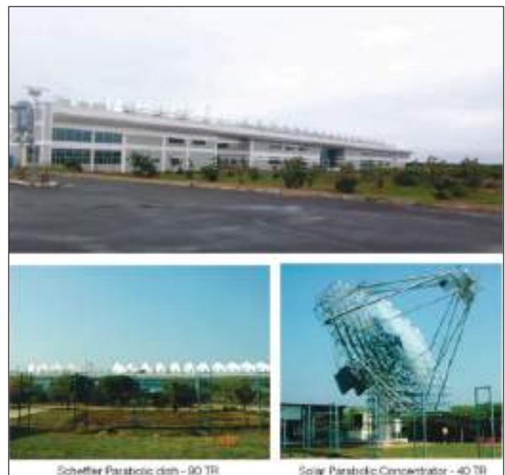
Fig. 5: Solar Parabolic Concentrator Generating Heat at 180 Deg C
