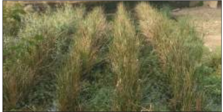
Fig. 4: Wetland Constructed to Convert Sewage into Clean Water
